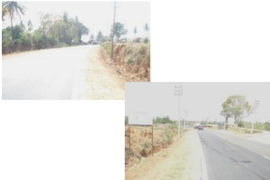
View of the Access Road - National Highway -207
